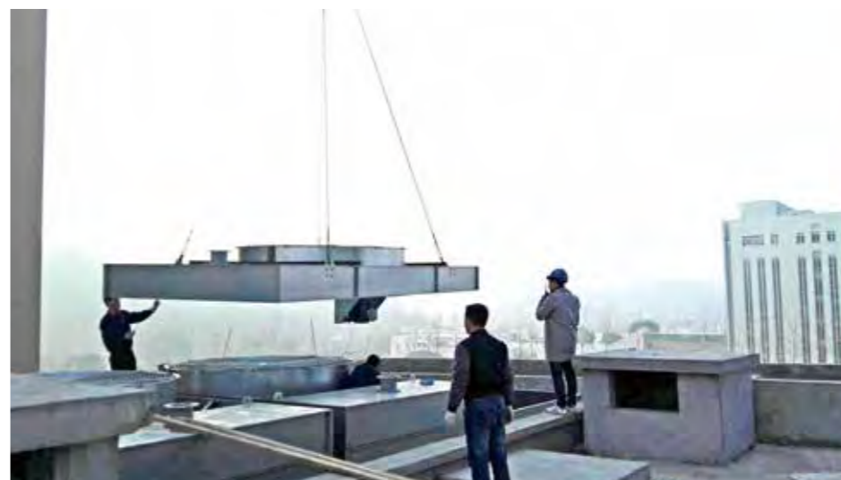
现场安装 Fabricating at Project Site
